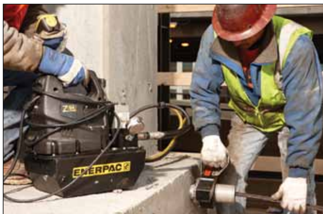
◀ The hydraulic PocketShear® makes quick and easy work of shearing tails on this elevated slab.
